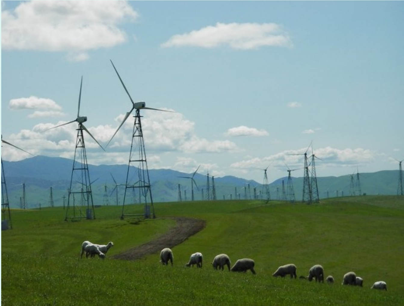
Dual land use: Rio Vista Wind Farm, California
