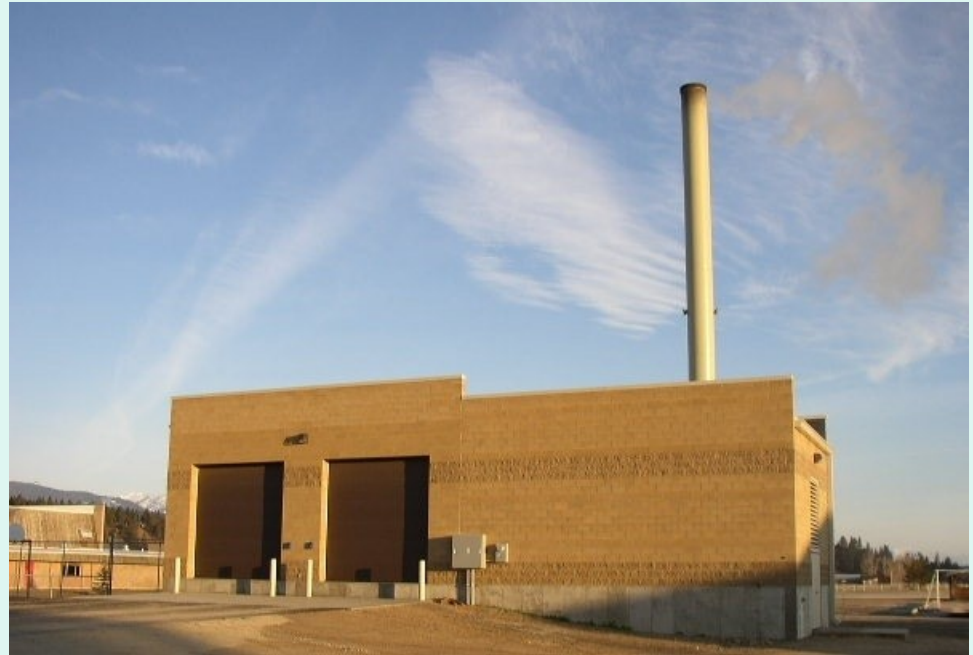
Biomass boiler at Darby Schools
