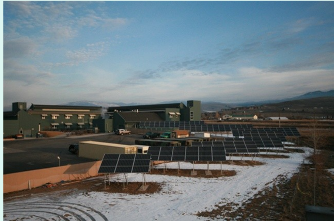
50 kW solar system in Missoula (Oasis Montana)
