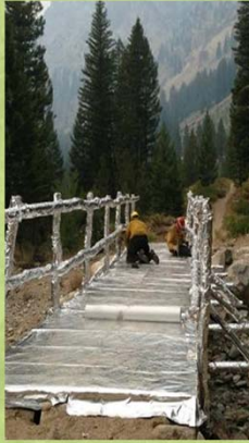
Structure protection - Wrapping a bridge
