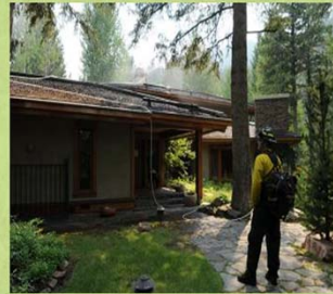
Structure protection - sprinklers and hose on a house
