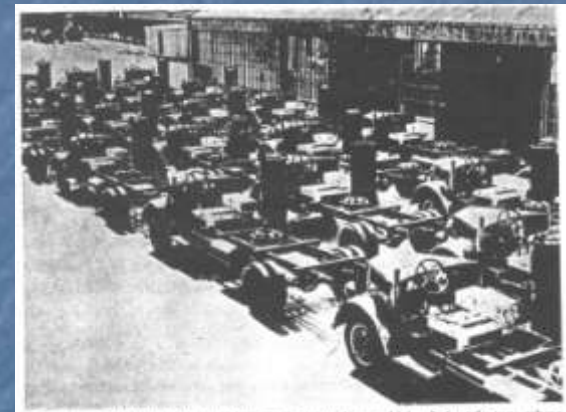
Germany, about 1943. Mass production of gas producer vehicles, Inbert factory, where some 500,000 gas producers were manufactured during World War II. (E. E. Donath)
