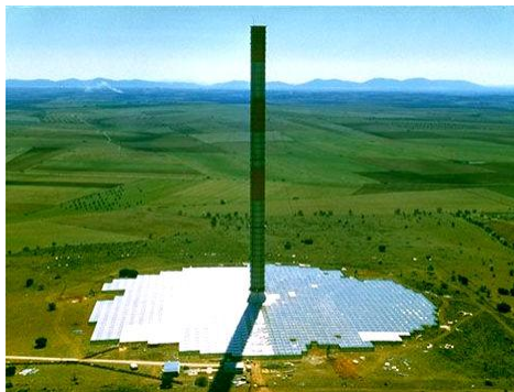
Figure 1 The small-scale pilot Solar Tower plant constructed in Manzanares Spain consistently generated 50kW. It operated between 1982 and 1989. (© 2001-2005 EnviroMission Ltd; RISE)
