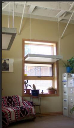
Office with daylight from Light Shelf
