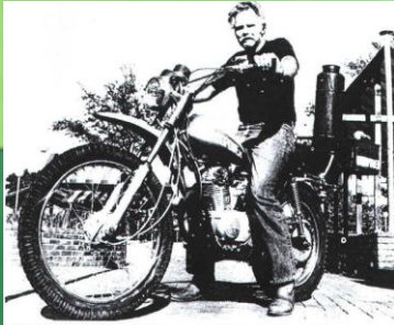
Gainesville, Florida, 1981. The tiny generator that powers this wood-burning motorcycle was constructed at the University of Florida out of a fire-extinguisher casing. The vehicle gets 70 km per kg of wood (20 miles per lb). (Glow Photo by Barbara Hansen)
