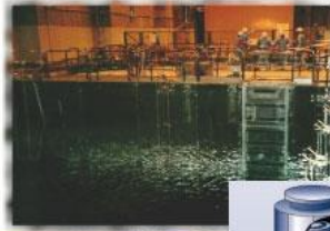
Fuel Rod storage pools
