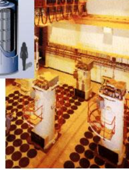
Loading silos with canisters containing vitrified high-level waste in UK, each disc on the floor covers a silo holding ten canisters
